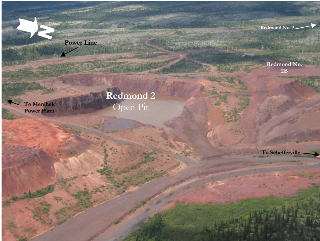
Figure 9: Air View of Redmond 2 Open Pit and Redmond 2B stripped area
