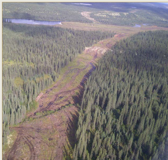
Aerial view – Houston Deposit. Access road tree clearing complete
